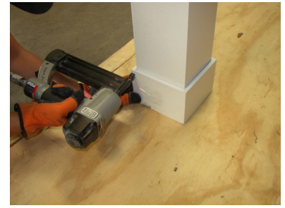
12) Fasten joints on base with pin-nails.
