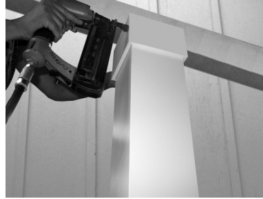
14) Install cap, repeating steps 11 and 12.
