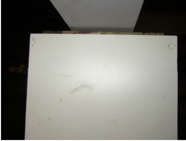
13) The TOP of the shaft should NOT be fastened to the post and there should be at least 1/2" gap to allow expansion (see step 2).
